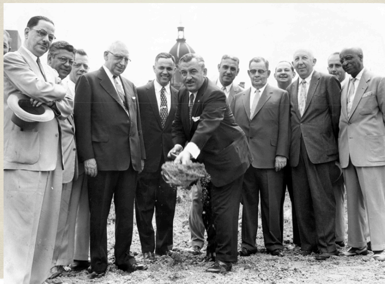
Broadway Project 1956 Breaking ground for a dormitory for medical students
